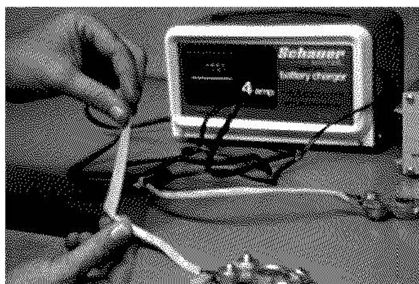
Figure 6. Wrapping the two negative leads together, into a single cable to the negative battery terminal (the positive leads have already been wrapped).
